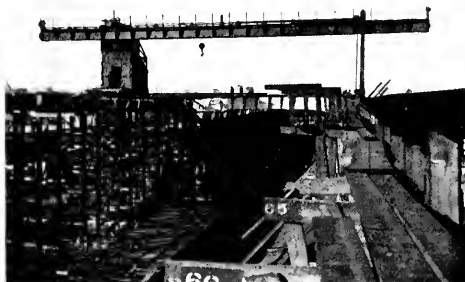
10-ton shipyard gantry crane at the American Shipbuilding Company's yard, Lorain, Ohio.
